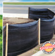
DeWitt Silt Fence
