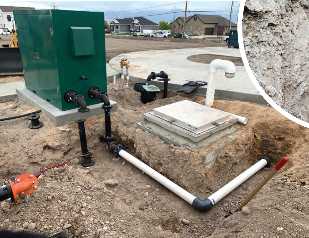
Working with two water sources was complicated, but having a detailed design and supportive representatives helped the team develop the creative solution needed. Using two float sensors let the system switch between groundwater and a culinary source, saving the city on water use. Photos: Tony Beckett
