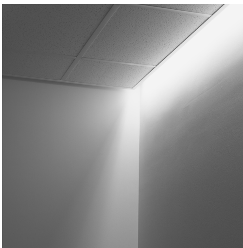
Typical Perimeter Light
